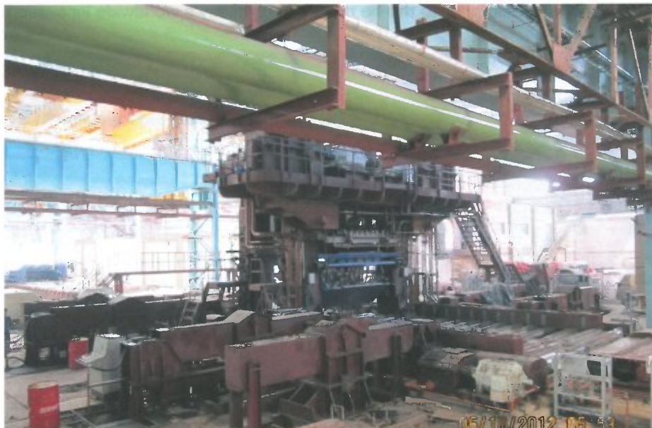
Hindalco hot roughing mill installation in progress at Hiralud, India.
